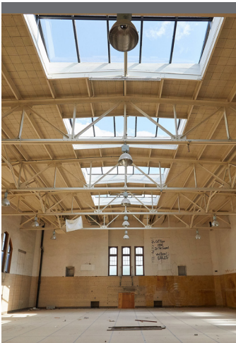
One of the gyms in Wittich is being stripped of its athletic gear, but the skylights will be kept for the remodeled office interior.
