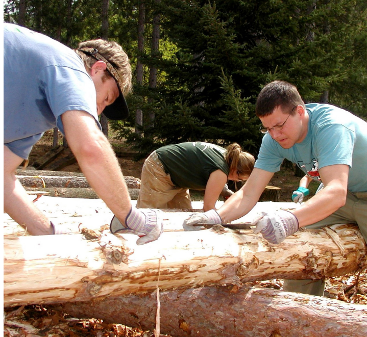
Recreation management students shave pine logs that were used to construct the Leopold Center near Baraboo, Wisconsin.
