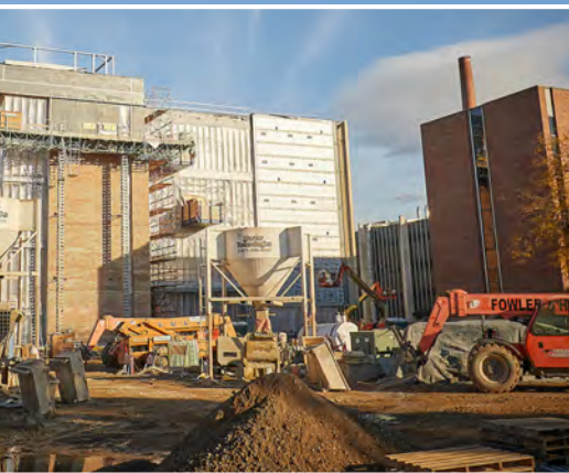
A view from the west side construction site project in October 2017.
