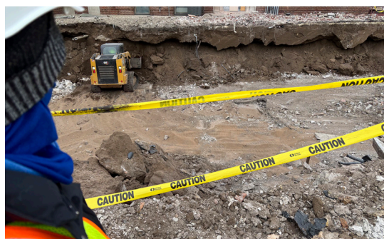
MVAC staff monitoring construction in January.
